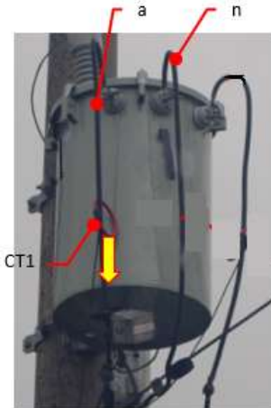
1 Ph, 2 Wire Configuration Fig.38
